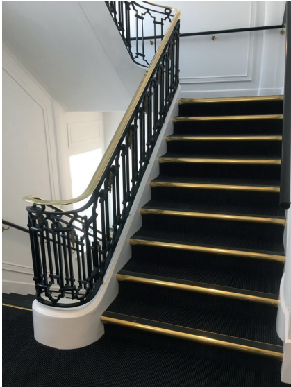
HN7 Gold Mirrorreflect stair nosings were used on a staircase at The Astor Court Hotel in London pics (above)
