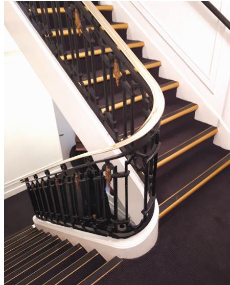
HN7 Gold Mirrorreflect stair nosings were used on a staircase at The Astor Court Hotel in London pics (above)
